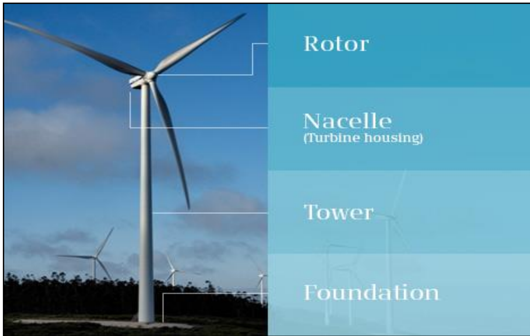
Plate 4-1 Wind Turbine Components
