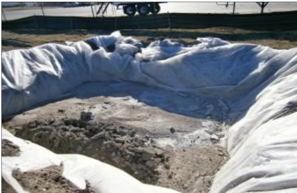
Plate 4-6 Concrete Wash Out Area
