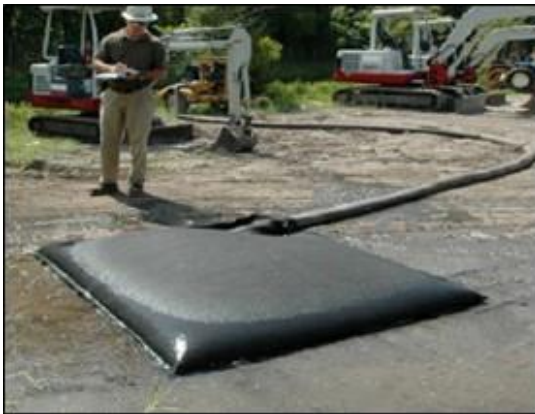
Plate 4-7 Silt Bag under inspection
