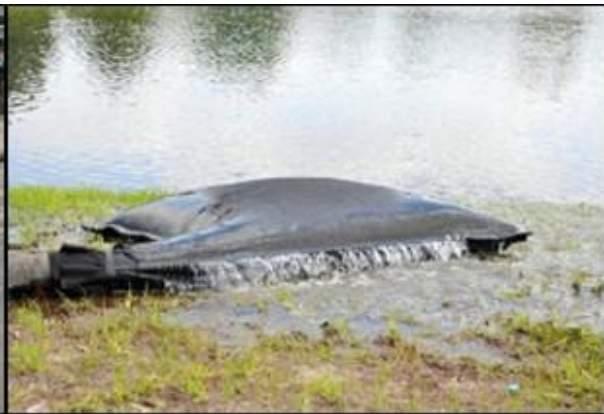
Plate 4-8 Silt Bag with water being pumped through
