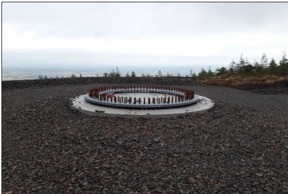
Plate 4-3 Finished Turbine Base
