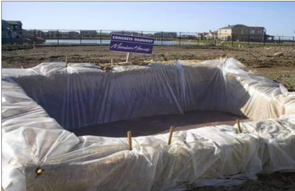
Plate 4-5 Concrete washout area
