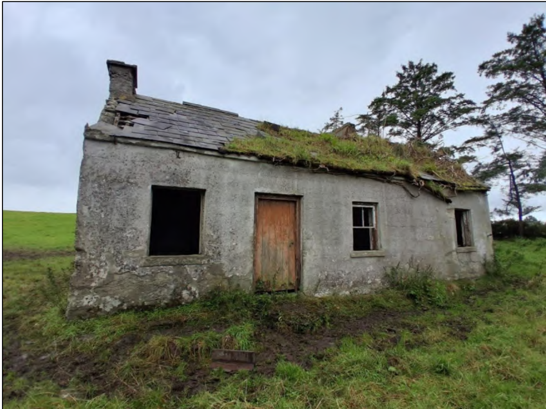
Plate 4-4 Existing Derelict Structure to be Demolished
